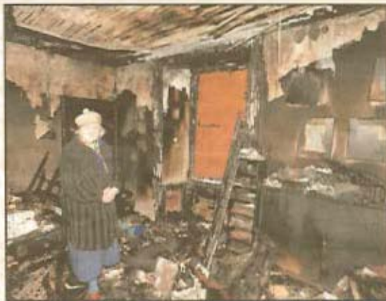
GUTTED: Jennefer Tobin surveys the damage to her study after her premises were hit by fire.
